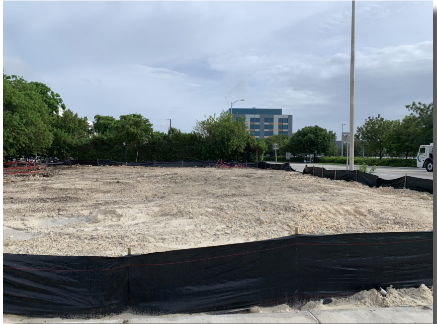
Above: The site of our future headquarters after demolition.
